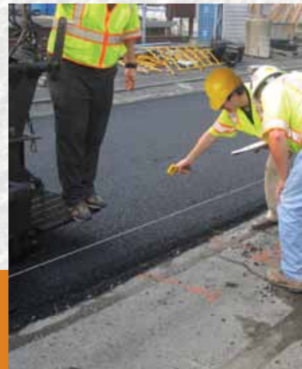
These FHWA researchers are documenting the temperature of a pavement mixture as it is being placed.
